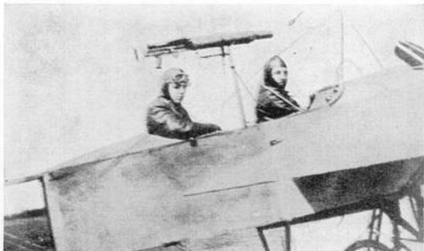
A standard Bleriot monoplane of 1914, showing the unusual method of mounting the Lewis gun. This is what might be called a "tripod mounting."
